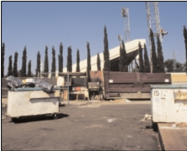
Site of Fire/Life Safety Training Center is currently the trash compactor yard.
