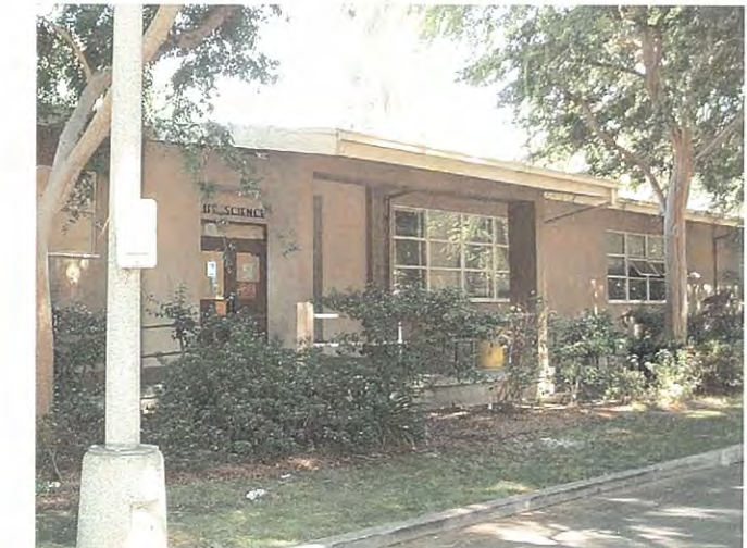
Single Story Instructional Building
