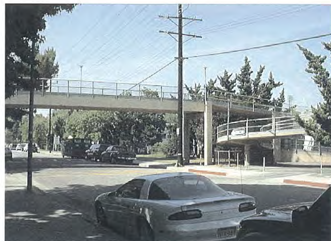
Closed Pedestrian Bridge on Ethel Avenue
